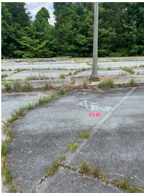
Location B-08 facing northeast
