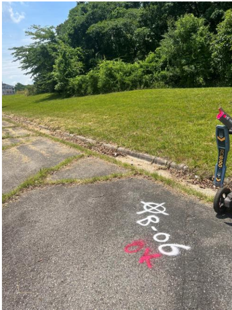
Location B-06 facing northwest
