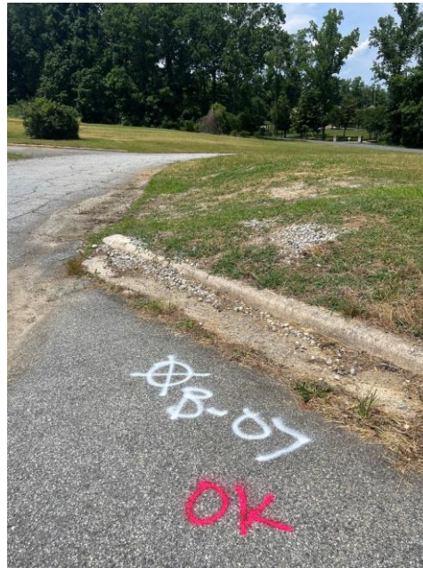
Location B-07 facing northeast
