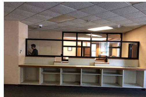
Interior - Administrative Offices
